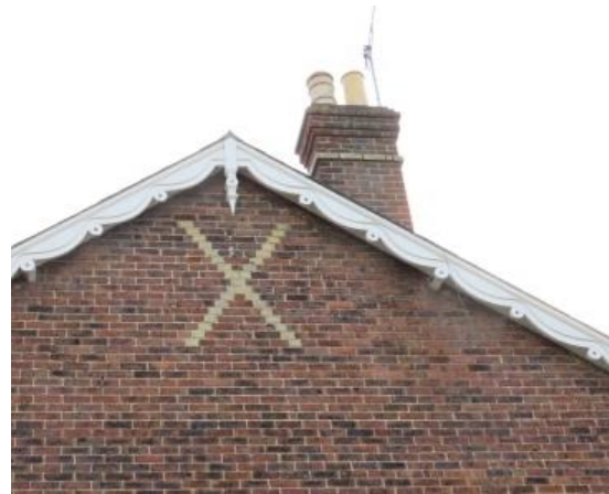
Brick and eaves detailing
