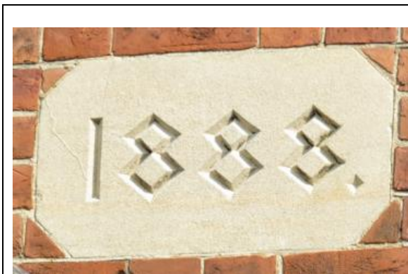
Date stone above the entrance to the Wesley Centre
