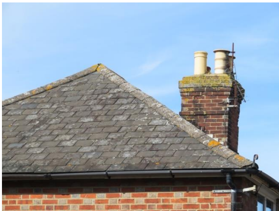
Roof tiles evident in central Paddock Wood
