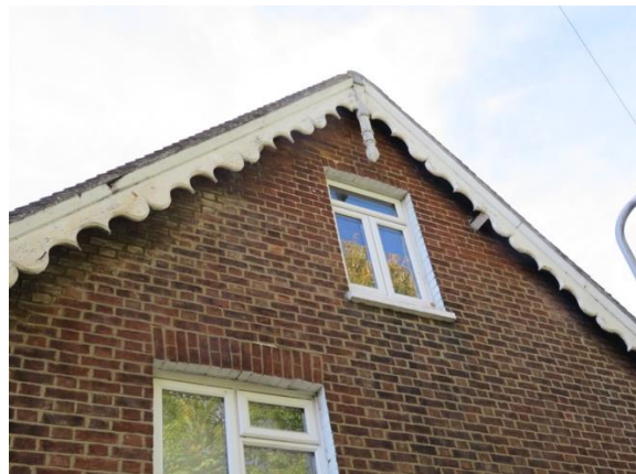
Eaves on Victorian buildings
